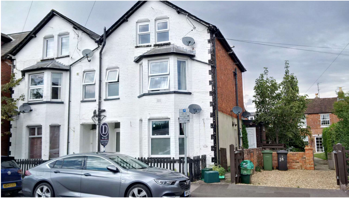
View of 34-38 Craven Road from Craven Road (looking north)
