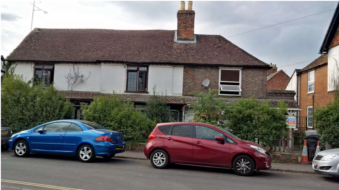
View of 1 & 3 Kennet Road from Kennet Road (looking West)
